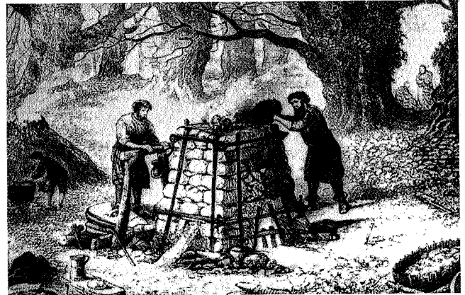
2-10. Typical pocket, or "testing" furnace, for testing the ore before investing in a full-size blast furnace stack. Note the foot-operated bellows at left (Fisher 1949:18).
