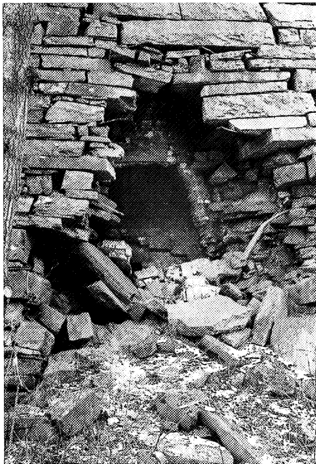
2-17. Massive breakdown of the Forest Dale stack conveniently exposed the in-wall and furnace lining for study, but also accelerated further deterioration in 1990.
