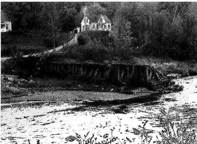
2-42. Although many mill dams were made of stone, others, such as this washed-out artifact in the Ottauquechee River at Bridgewater, were made of wood with a stone base.
