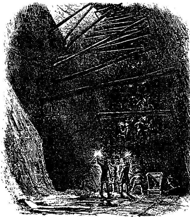
3-14. Typical view inside a mine, showing timbers that kept the walls from collapsing into the workplace (Orr 1860:588).
