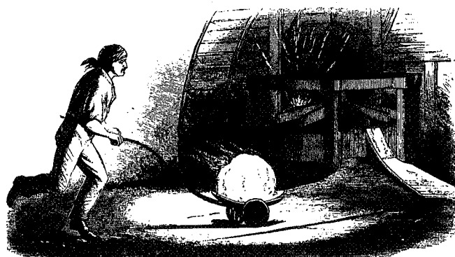
2-34. Transporting a red-hot bloom from the puddling furnace to the hammer, where the bloom was worked into a manageable shape (Chapin 1860:159).
