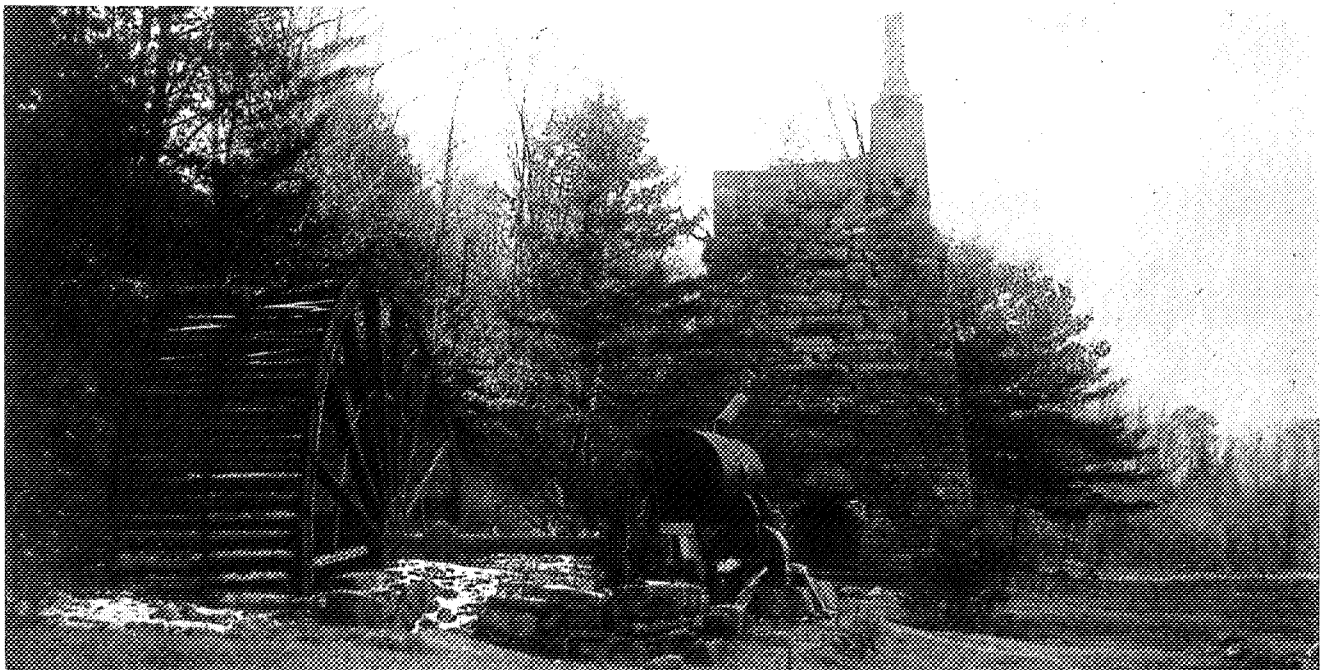
2-23. Ca.-1915 view of waterwheel, blast machinery, and heating ovens (top of the furnace) at Forest Dale (courtesy Vermont Division for Historic Preservation).
