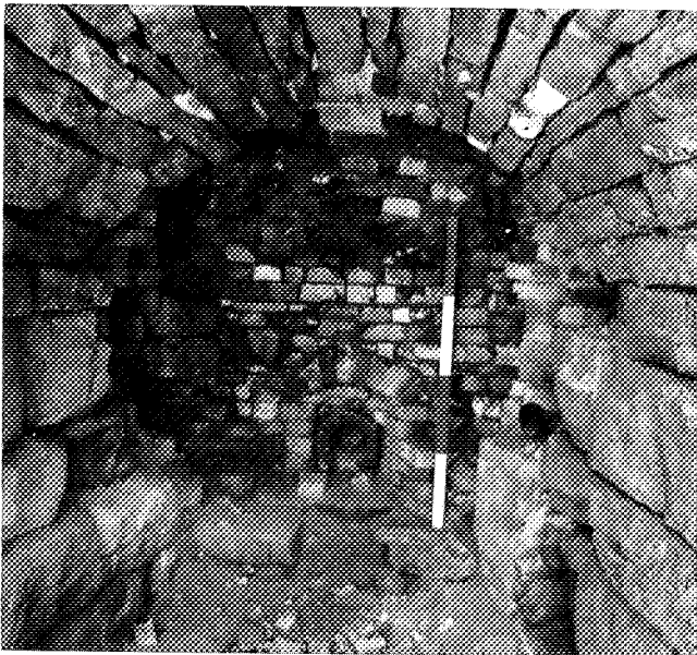
2-26. Broken end of a bustle pipe (right) and the tuiere (center) at the Forest Dale furnace (courtesy Vermont Division for Historic Preservation).
